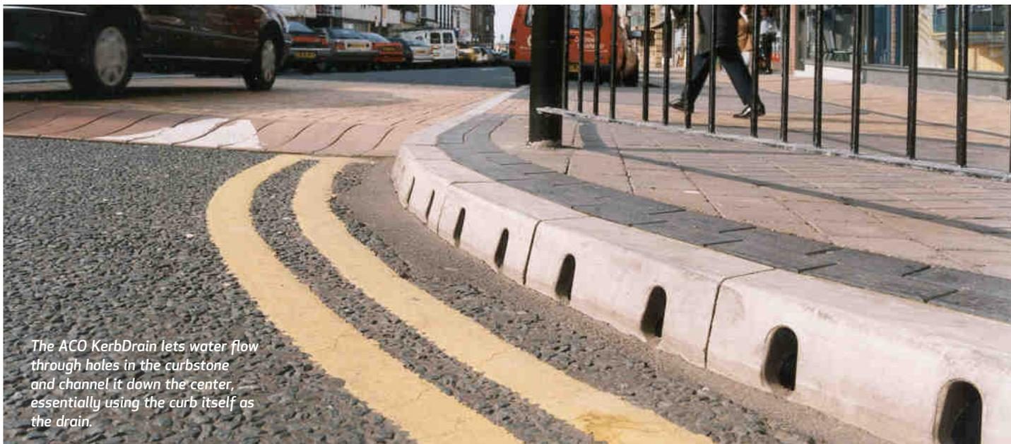
*The ACO KerbDrain lets water flow through holes in the curbstone and channel it down the center, essentially using the curb itself as the drain.*
